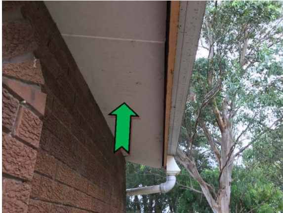
Photo 1. Exterior, west elevation, eaves – non asbestos-containing fibre cement sheeting.
