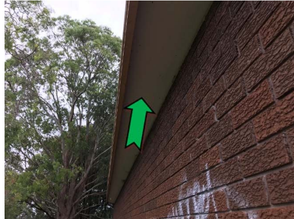
Photo 2. Exterior, east elevation, eaves – assumed non asbestos-containing fibre cement sheeting.
